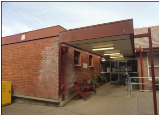
Figure 3.30 The entry which is located at the junction of the earlier Jennings Building (c. 1956) and the addition (c. 1976) has a modern steel framed canopy.
