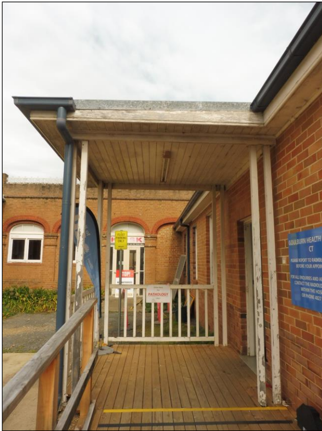
Figure 3.14 The existing external entry. Varying brickwork on the façade indicates additions and infill of the former verandah spaces.
