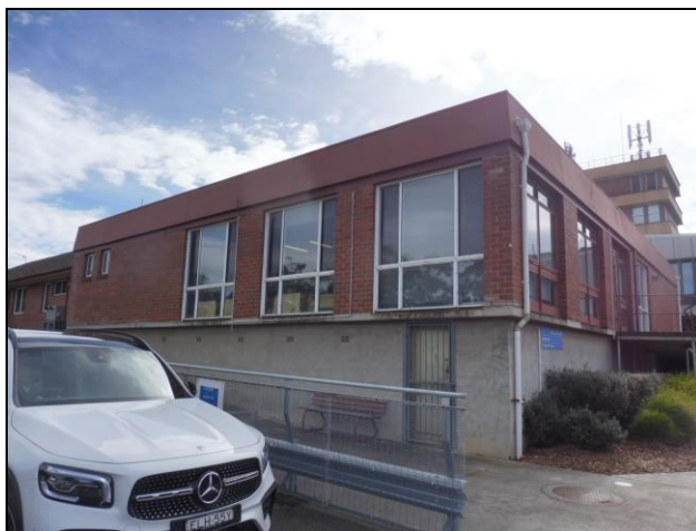
Figure 3.26 The building is a modern brick structure on a concrete base with flat roof clad in metal sheeting and aluminium framed windows and doors.
