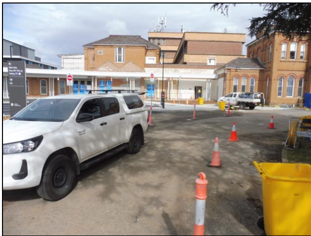
Figure 3.6 The main building comprises three, two storey pavilions and associated single storey wings and additions which extend from the central pavilion. The original pavilions are face brick with hipped roof clad in tiles and contrasting brick and stone details, timber framed windows with round and flat arched heads and timber doors.
